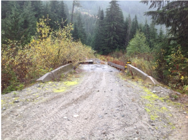
Approach from Right Bank when facing downstream
