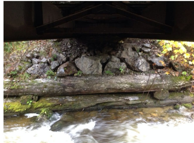
Right Bank Abutment when facing downstream
