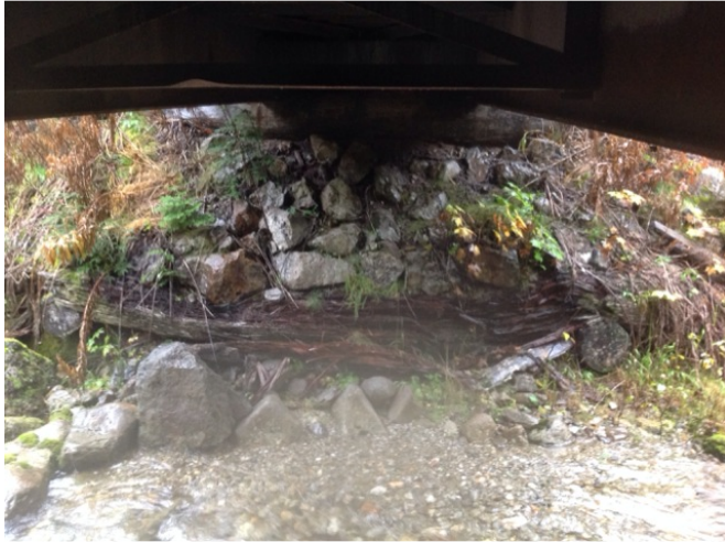
Left Bank Abutment when facing downstream
